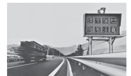
The world's first road weather information system installed on the Tomei Expressway used an illuminated board to automatically display traffic warnings (1969)
