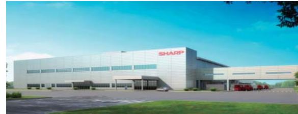
Plant No. 2 at SOCC began operations in April 2012
