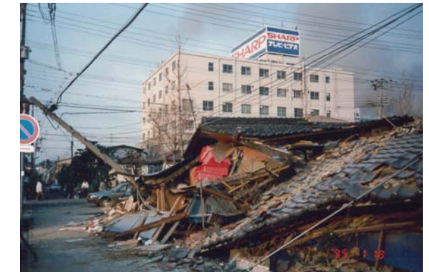
Devastation around the Sharp Kobe Building
