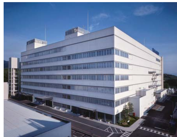
The LCD plant in Tenri, where large, high-quality TFT LCDs were efficiently produced
