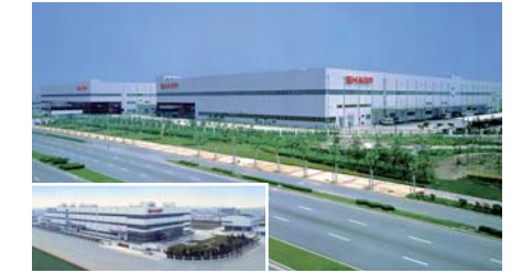
Manufacturing company SSEC in China
