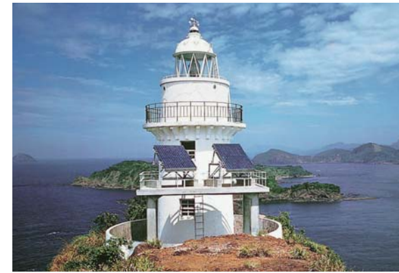
The Ogami Island Lighthouse is powered by Sharp solar (photo courtesy of Japan Coast Guard)
