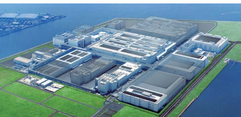
Aerial view of Green Front Sakai (as of 2011). The area within the dashed lines and the rooftop solar panels are conceptual renderings showing the appearance when finally completed.
