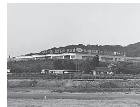
The Hiroshima Plant, a dedicated radio factory (1967)
