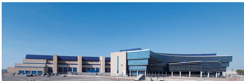
Thin-film solar cell plant in Italy (scheduled to start production at the end of 2011)
