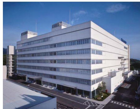
The LCD plant in Tenri, where large, high-quality TFT LCDs were efficiently produced
